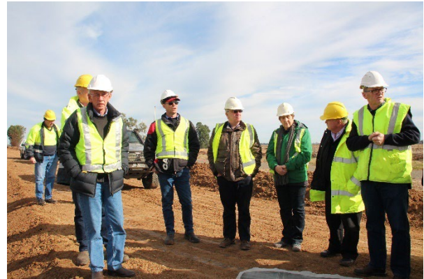
Bruce Brown, CICAL staff, former directors and former CEO inspecting infrastructure upgrades.
